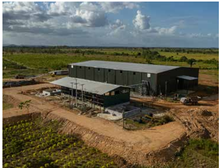
Top to bottom; Packaging cocoa after the high volume bean sorter process; Main area of the new processing center; Aerial view of the new processing center.
